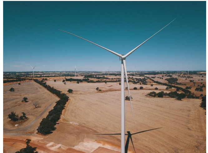
FRWF1 is currently in the generator performance testing phase
