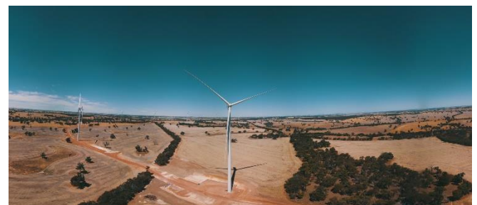
All 18 turbines at Flat Rocks Wind Farm Stage 1 have been installed
