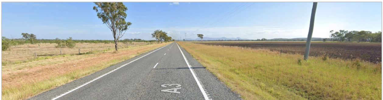
Figure 4.6 Burnett Highway Facing North
