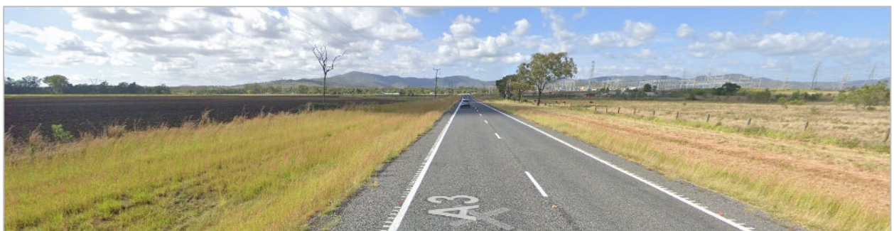
Figure 4.7 Burnett Highway Facing South
