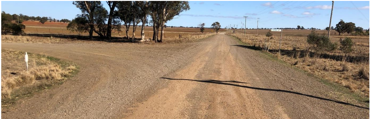
Figure 13: View West down Back Trundle Road from McGrath Intersection
