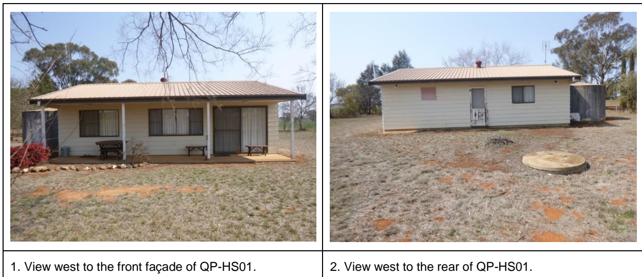
Figure 10-2: Photographs showing an overview and details of QP-HS01.
