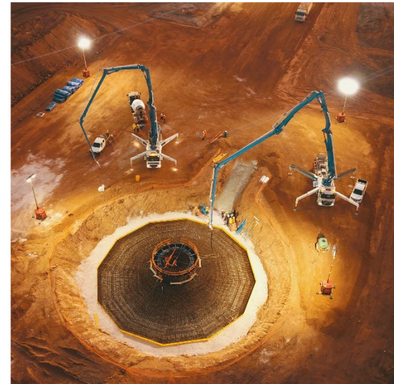
Concrete pour of a wind turbine foundation underway.
