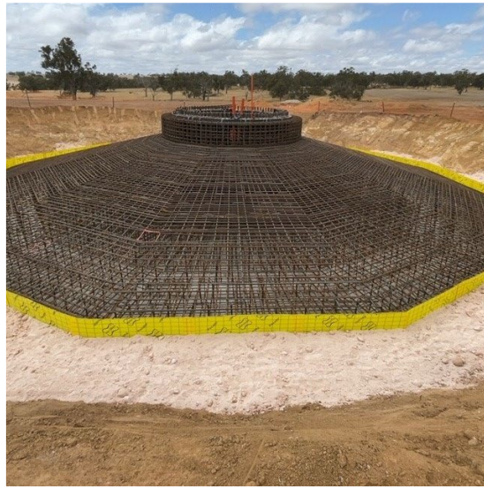
Wind turbine foundation ready for the 'concrete pour'
